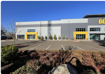
1980 SE 4th Avenue, Suite B Braber Equipment Building, Canby OR SF Leased: 37,500 SF
